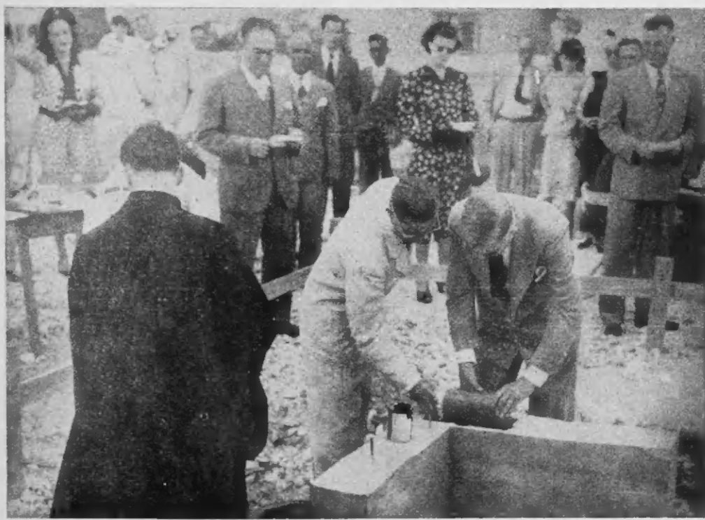
On Easter Sunday the cornerstone of the Protestant Congregation Church of Aruba was laid in Oranjestad. Members of the Church look on as Addison W. Croes (right) lays the cornerstone of the building. In the center is Lt. Gov. L. C. Kwartzs who, with Mr. Croes, placed a scroll in the cornerstone, and at left, with his back to the camera, is the minister, Rev. J. J. van de Wall. The church was designed by architect Jan Nagel, of the Construction Company Aruba, and is being built under his direction. It is estimated that the building will cost Fls. 225,000 and require 18 months to finish. It is being built near the site of the old church and will have a seating capacity of 300 persons. Money to build the church is being raised by the church council with the assistance of the finance committee. Members of the council are Rev. van de Wall (chairman), J. H. Beaujon (secretary), Godfried Croes (treasurer), C. H. G. Eman, J. R. Beaujon, E. O. Frigerio, and E. O. Lampe.
